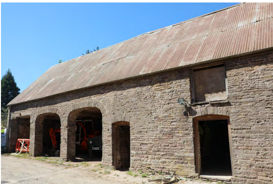
Cart shed with granary over and stabling with loft over Tŷ-Mawr Farm, Llangasty. Photo © Sam Hale
