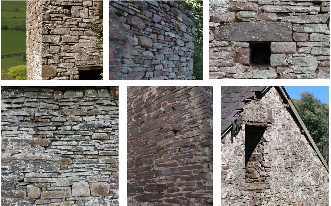
Examples of rubblestone across the National Park. Clockwise are the sandstones of the Dyffryn Crawnon, multi-colours of Pontsticill, grey greens of Llanfrynach, limewash remains at Llanddeusant, mixed purple-maroon sandstones near Blwch, olive-green and pale sandstones of Ystradfellte. Photos © Sam Hale
