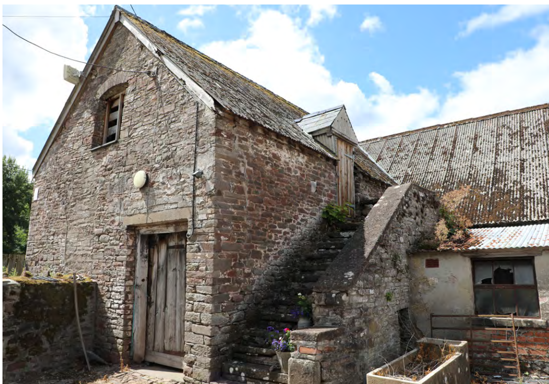
A large first-floor granary at Pencelli Court, marked by shutters and with a hole for unloading grain along a chute. Photo © Sam Hale
