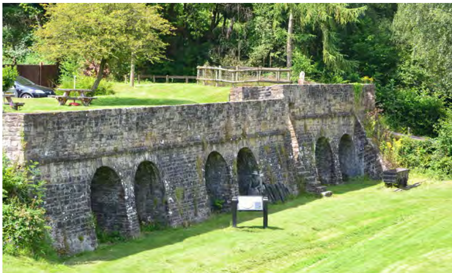
Industrial lime kilns at Goytre Wharf alongside the Monmouthshire and Brecon Canal. Photo from Geograph, © David Martin and licensed for reuse under Creative Commons Licence
