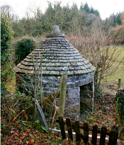
A circular ‘beehive’ pigsty at Upper Llanover. Photo © Clywd and Powys Archaeological Trust 21762
