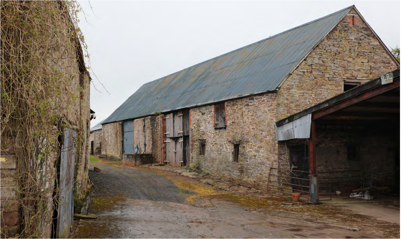
Penyrwylod farm on the road to Trewalkin, Talgarth. A farmstead with buildings dispersed along a route – the house a c.17th century longhouse derivative with later farm buildings including this combination barn with two threshing doors. Photo © Sam Hale
