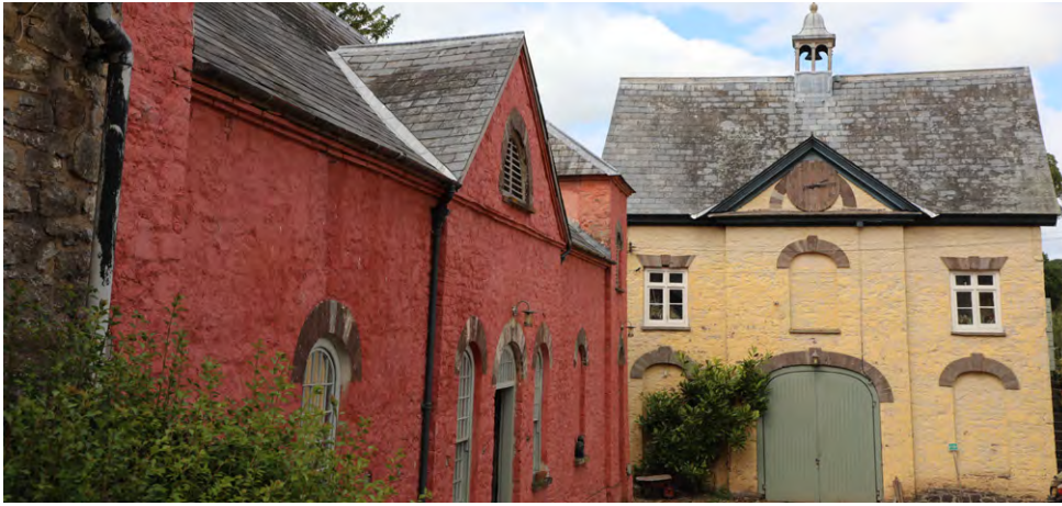
The very fine late 17th or early 18th century lofted stable range at Penpont with coach house, restored with colourwashed walls in c. 2000. The formal facade of the stables has two outer bays treated as pyramid roofed pavilion towers and the centre three bays pedimented and slightly projected. Photo © Sam Hale
