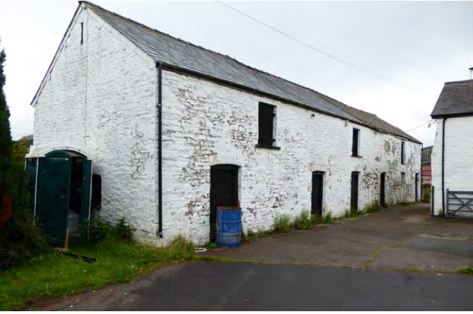
A two-storey cow house with its row of doors to stalls and hay loft, near Crai in the Western Usk Tributaries. There are timber-framed examples of these dating from the late 16th century along the Border Counties, but in the National Park these stone-built structures are all 19th century. No earlier examples have yet been identified. Photo © Jeremy Lake
