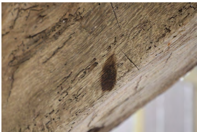
A burn mark on a principal rafter in Lower Trewalkin longhouse, Talgarth. Photo © Sam Hale
