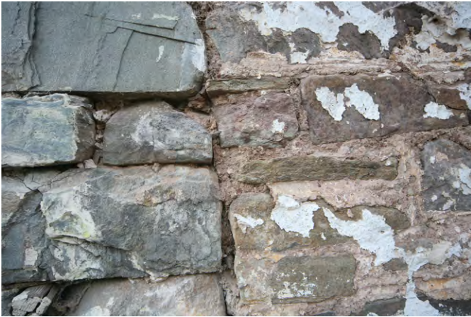
Raglan Mudstone - silty mudstones with calcretes and sandstones occasionally mixed in with limestones laid in a hot mix earthen mortar with quicklime. There are traces of copperas or deep ochre limewash with later synthetic masonry paint over. Photo © Sam Hale
