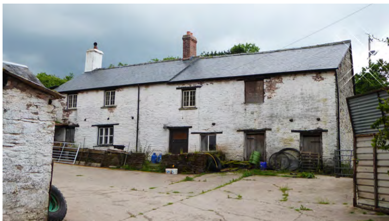
A linear farmstead at Cwm to the east of Talgarth (Wye Valley Foothills). It was remodelled early in the 19th century, with a loft above housing for cattle and horses, and additional farm buildings then made an overall U-shaped plan. Note the wide doorway placed to the right of the central chimney stack, which offers a hint that this building may have developed from a longhouse with a single entrance for people and cattle into a wide passageway. Photo © Jeremy Lake
