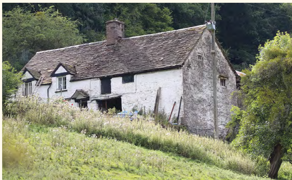
The siting of this 16th century longhouse in the Black Mountains is typical, with its cattle housed in the downslope end. It was remodelled in the early-mid 19 th century when the original cross-passage doorway was made into a barn door. Photo © Sam Hale
