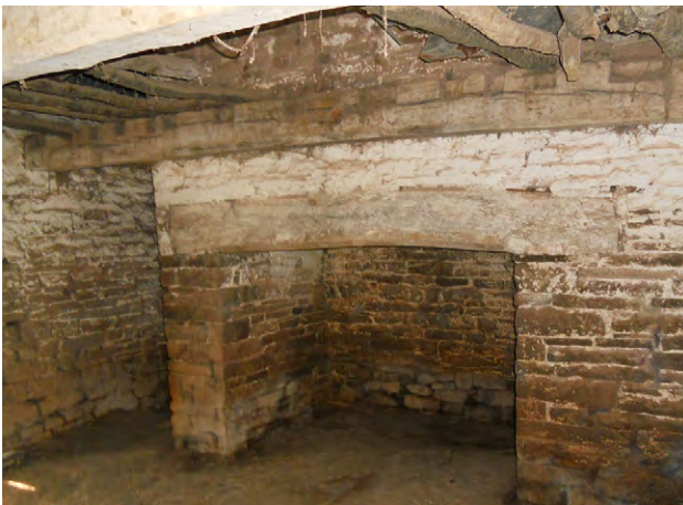
An open fireplace and the remains of a bread oven in a bakehouse. Photo © Sam Hale
