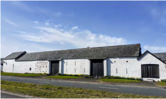
A large threshing barn with two threshing floors at Cefn Brynich, alongside the A40 in the Usk valley to the east of Brecon. Photo © Sam Hale
