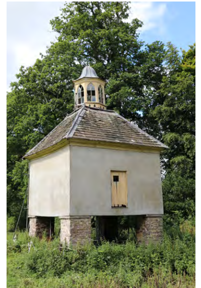
The superb dovecotes at neighbouring Abercamlais and Penpont. At Abercamlais the extraordinary 18th century stone dovecote sits on a bridge over the Camlais, the base formerly a privy with effluent carried away by the brook into the Usk. At Penpont the 18th century timber-framed dovecote is raised on stone piers, with a first floor chamber and dove access through tiny openings in the glazed cupola. Photos © Sam Hale
