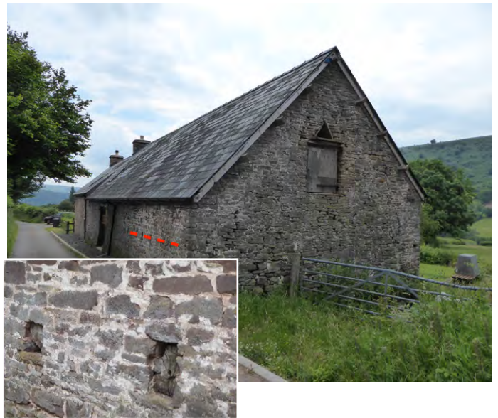
The Black Mountains has some of the earliest evidence for cattle housing in Wales or England. To the top left is the late 17th or early 18th century cow house at Tyn-y-Llwyn, Partrishow (see page 30). Like other high-status examples of this date, it has outer entrances for cattle. To the right is a barn of a similar date, with beam ends indicating the presence of a loft floor. Photo © Jeremy Lake
