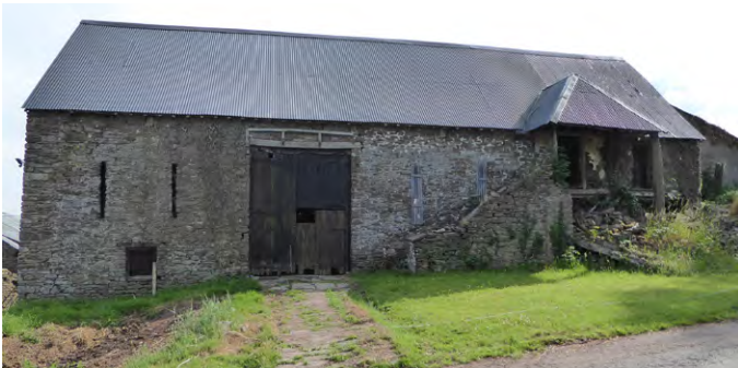
A very large combination barn at Tre-fedw, on the eastern fringe of the Black Mountains. This may date from the early 18th century, and apart from the threshing barn with its double doors has a cow house to its lower (left-hand) end with gable-end doorways, and steps rising to a granary set above cart sheds to the right. Photo © Jeremy Lake
