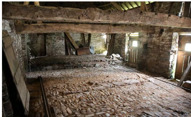
A cobble floor to a cowhouse. Photo © Sam Hale
