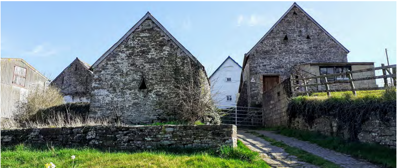
A parallel linear downslope group at Bwlch. The 17th century farmhouse originally had a beast house at the lower end, later converted to an extension of the dwelling in the early 20th century. The farm buildings are 18th century and consist of a barn at the upper end and a cow house below under a separate, lower roof. Photo © Sam Hale
