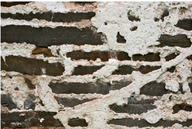
Sandstone laid in earthen mortar with a very lime rich parging finishing mortar for protection. Photo © Sam Hale
