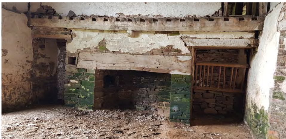
Conversion of a farmhouse to agricultural use has here left the open fireplace and a beam from the upper floor. Photo © Alice Thorne
