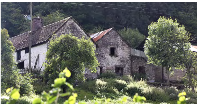
Coed, Vale of Ewyas - A 17th century detached kitchen (middle) with accommodation over which became an agricultural outhouse when the longhouse (left) was improved by the Llanthony Estate in the early/mid 19th century. It had a cart shed added to the uphill end at this time. The interior of the ground floor retains its fireplace and copper, the first floor served as accommodation. Photo © Sam Hale
