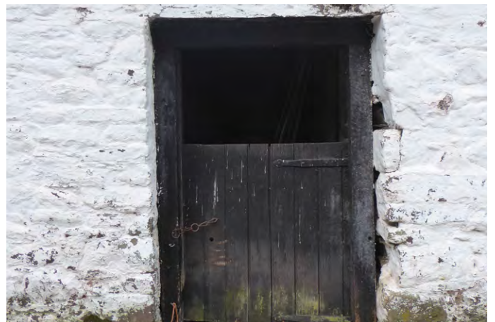
A plank door with strap hinges made in the local forge, and set in a heavy pegged frame. Split level doors were commonly used. Photo © Jeremy Lake
