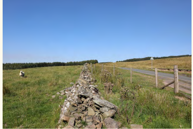
Christie's enclosing drystone walls, now collapsing. Photo © Sam Hale
