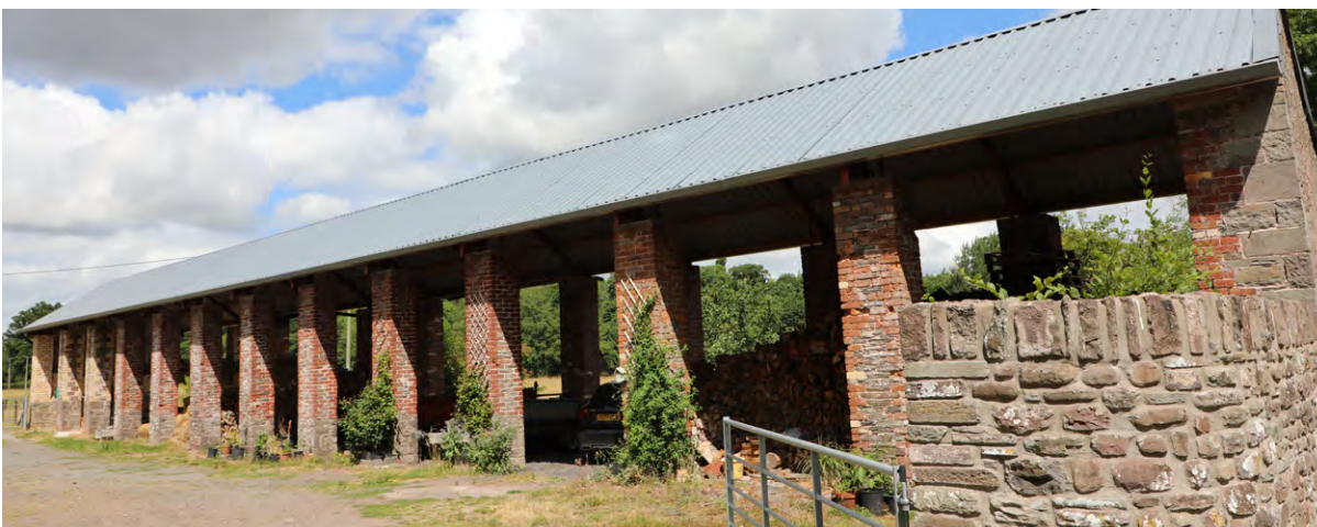
Huge 12-bay hay barn on brick and stone piers, Tŷ-Mawr, Llanfrynach. Photo © Sam Hale
