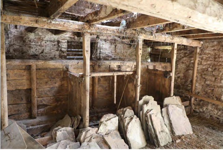
Interior with chamfered cow ties and feed passage, Llanigon. Photos © Sam Hale
