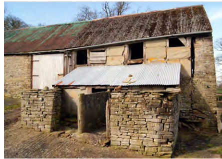
This is the most common type of pigsty, with covered housing opening onto a yard. Photo © Sam Hale
