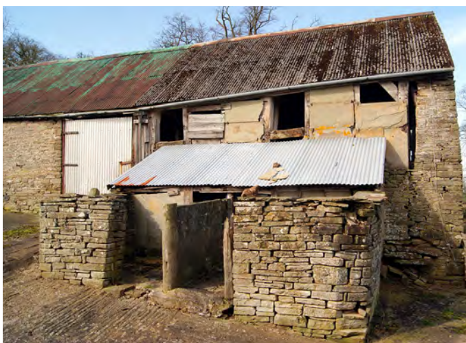
Surviving timber frame is rare. This 17th century framing survives from the rebuilding in stone of a barn in the Wye Valley Foothills. Note the use of massive flagstones pinned to the timber frame. Photo © Sam Hale
