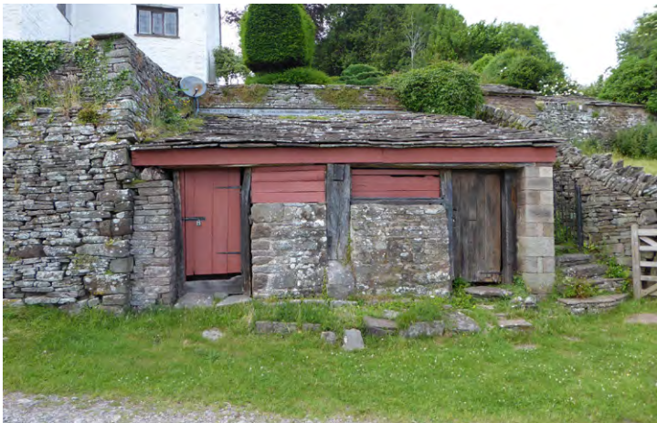
This former open-fronted shelter shed was converted into loose boxes in the mid-late 19th century, and was used to house bulls. Photo © Jeremy Lake
