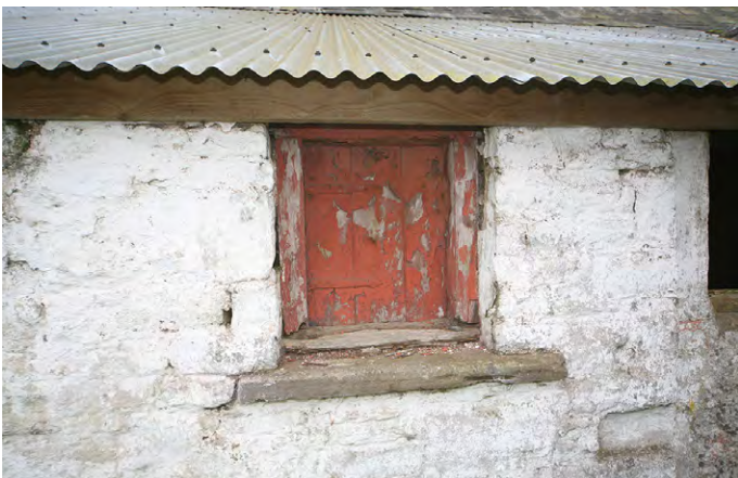
Wooden shutters were commonly used, and can now be rare survivals. Photo © Sam Hale
