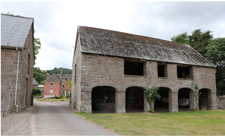
The large 5-bay lofted cart shed at Abercynrig (glimpsed behind). The cart shed contains a cider mill and press. Photo © Sam Hale
