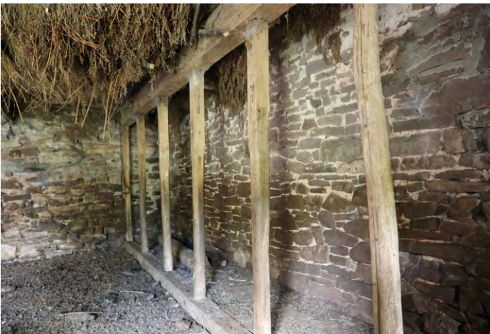
Simple single cow ties in a combination barn, Dyffryn Crawnnon – note the loft above supported with bundled poles of hazel. Photo © Sam Hale
