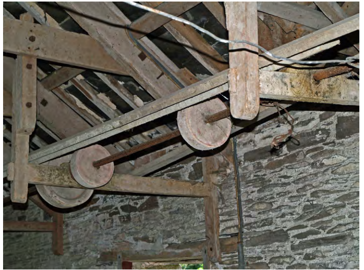
A belt drive and line shaft. Photo © Jeremy Lake
