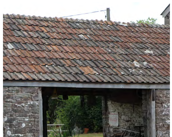
Double Roman Bridgewater clay tiles at Pencelli Court – possibly brought up the canal which runs alongside the farm to re-roof the barn. Photo © Sam Hale
