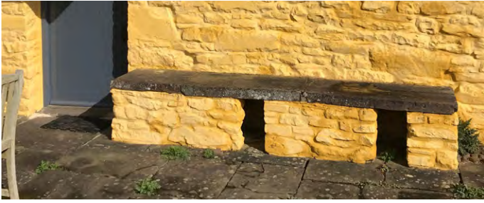
Gooseholes are commonly placed next to the back door of the farmhouse, as here. Photo © Sam Hale
