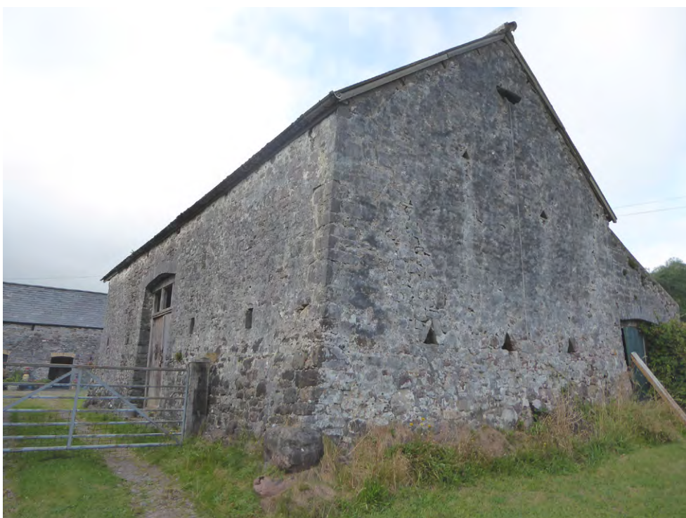
The barn at Rhongyr Uchaf, with a datestone of 1839 but with earlier footings visible in the lower courses of the masonry. Photo © Jeremy Lake
