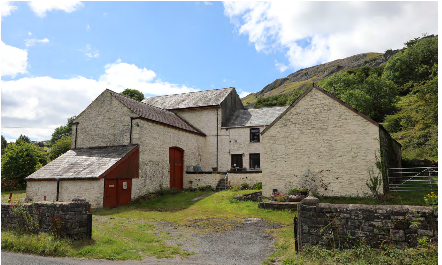
Gelli, situated south of Craig-y- Nos. A small quarry and limekiln were located just behind the farm range. The compact U plan range comprises a barn, lean-to cart house, cow house, and (just out of shot) two pigsties. Photo © Sam Hale
