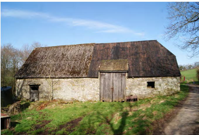
Combination barns with a lofted cow house at one end are a common feature, some examples dating from the late 17th century. An example (shown left) at Maestorglwyd in the Black Mountains was adapted from an early 15th century hall house, the earliest dated hall house in the Brecon Beacons. Photos © Sam Hale
