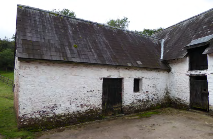
The wide doorway to this early 19th century or earlier building at Ynys-fawr in the Western Usk Tributaries may be indicative of it allowing access by oxen. Photo © Jeremy Lake
