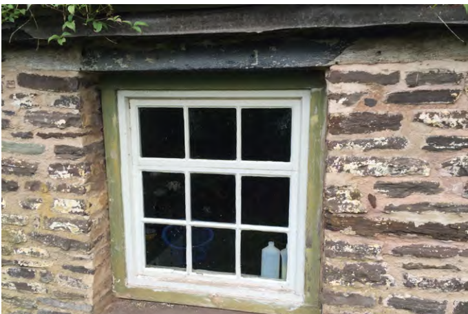
Particular to the area is the Brecon Hopper, a local window type commonly used between around 1870 and 1940 with a side-hung casement over a multi-paned sash or fixed window. Photo © Sam Hale
