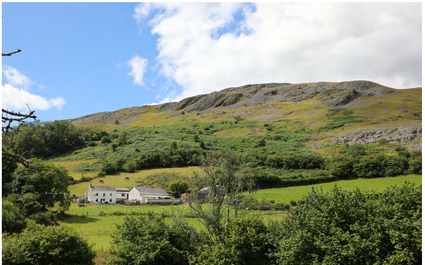
Pant-y-Wal, Craig-y-Nos – detached farmhouse and limewashed threshing barn set among later buildings set below Cribarth which has been extensively quarried and is criss-crossed by former tramroads. Photo © Sam Hale
