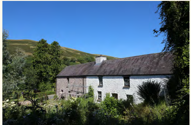
The Gorsddu linear range opposite which is a small combination barn/cow house. Photo © Sam Hale
