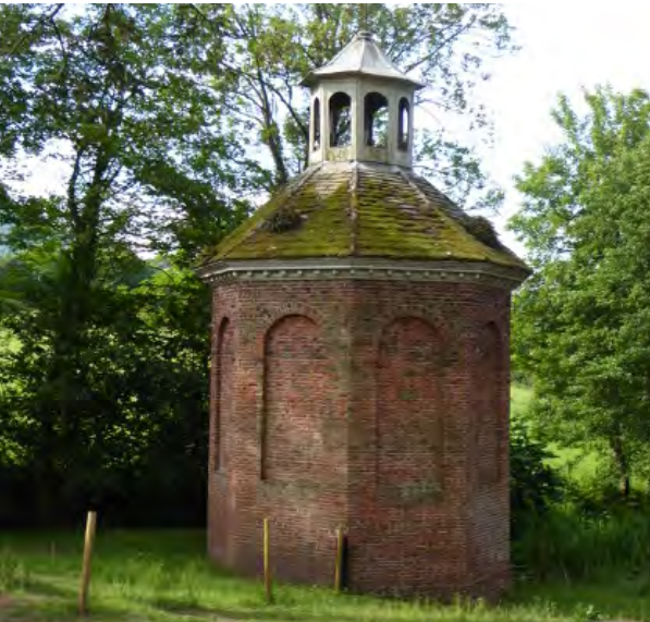
An unusually fine and brick-built late 17th century dovecote, probably built at the same time (1692) as the fine house it stands next to Trewyn on the eastern edge of the Black Mountains. Photo © Jeremy Lake
