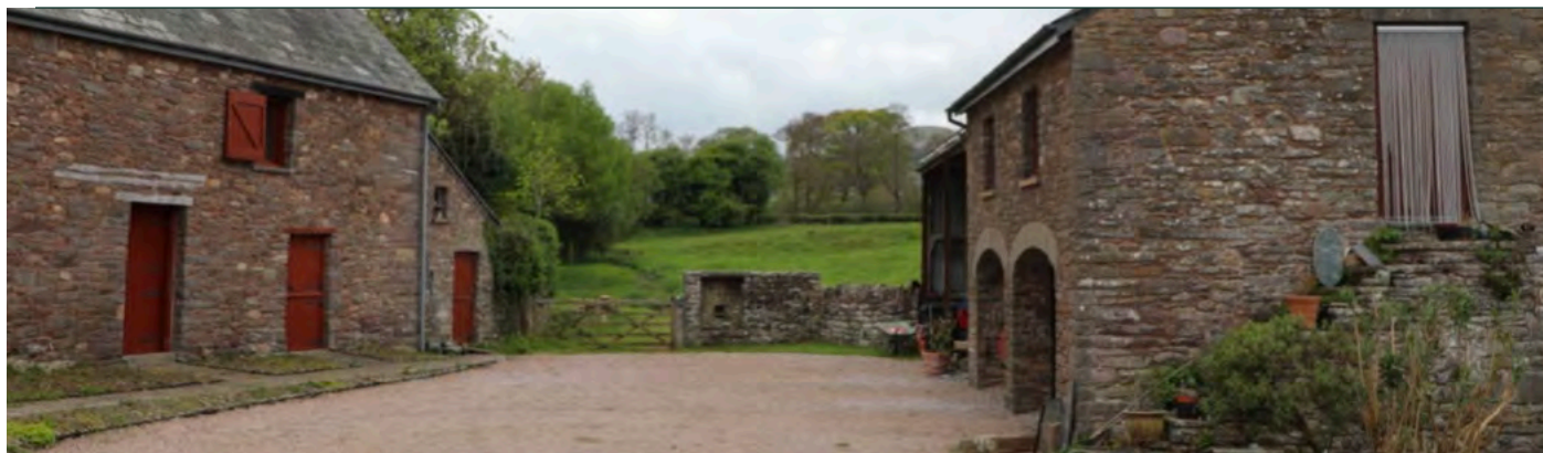
The 19th century additions of cow house and stables with loft over (left), and cart shed with granary over (right). Photo © Sam Hale
