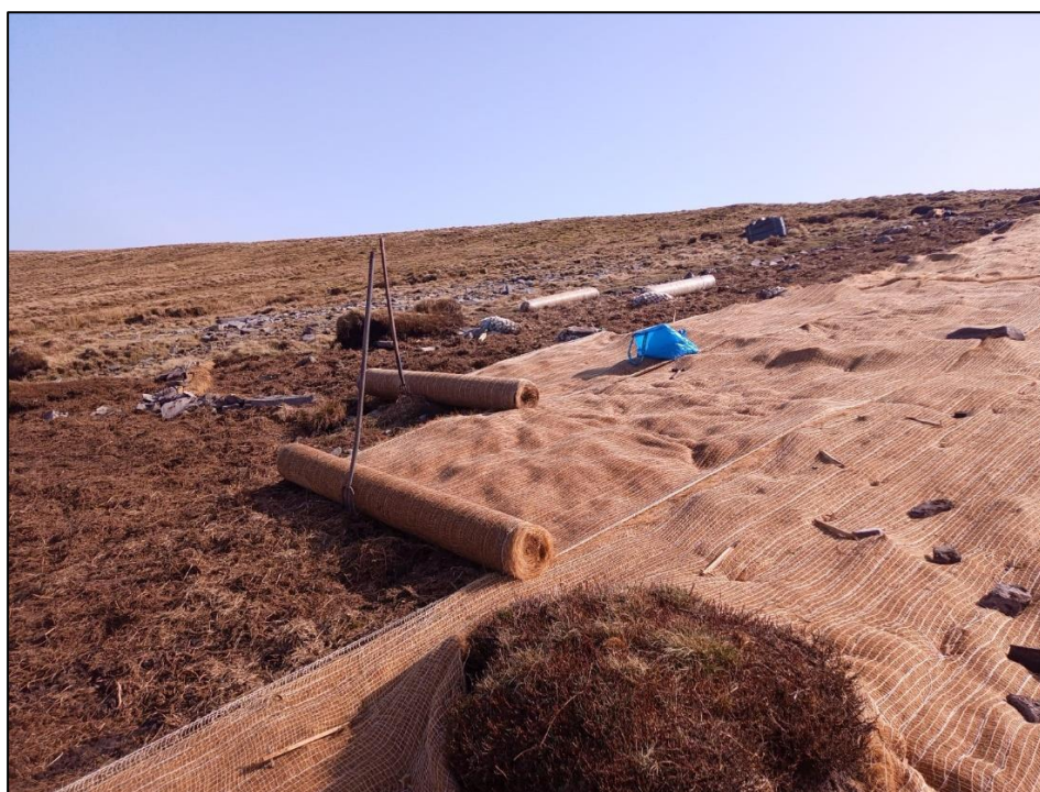
Photo: Peatland restoration at Pen Trumau – laying coir matting on top of heather brash
